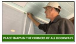
**STEP 3)** Attach the sides of your curtain panels with marine snaps. Begin by sealing all zipper doorways. Pull panels to edges and decide how much overlap you want on your sealing surfaces. The edge of the panel will extend slightly beyond the edge of your surface.
