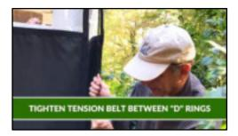
**STEP 2)** Strategically place L-screws and marine snaps. To seal the base of your curtain, you will create side to side tension at the base. The two main methods for sealing the base are strategically placing marine snaps in the bottom corners and placing belted ribs in free corners. Begin by placing L-screws in the corners to create tension.
