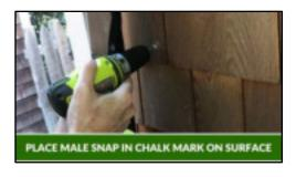
5 is a good number of marine snaps to place for applications under 8' tall. Place snaps every 12-18" depending on your wind conditions. Equally space snaps top to bottom. Snap each snap into place from the top and pull down to create vertical tension as you go. This vertical tension makes the webbing lay flat and creates a nice seal against the surface.
