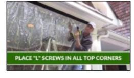
**STEP 2)** Hang your curtain by firmly pressing the loop-sided Velcro® strip sewn to the top binding to the hook-sided strip adhered to your surface. If you have surface gaps, you can under mount a wood strip. Place L-screws & marine snaps in the corners of all zipper doorways.
